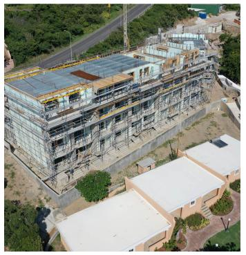
The project used ICFs for all exterior walls and demising walls to maximize energy efficiency and **sound attenuation** with the high R-value and STC ratings of Nudura ICF blocks. Steel reinforcement was incorporated into the insulated concrete form assembly so the resort will also be protected from seismic activity, tropical storms and hurricanes.
