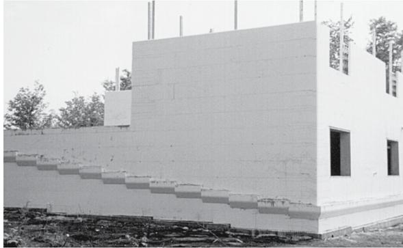
(152 mm), 8" (203 mm), 10" (254 mm) and 12" (305 mm), with an overall thickness of 9 1/4" (235 mm), 11 1/4" (286 mm), 13 1/4" (337 mm), 15 1/4" (387 mm) and 17 1/4" (438 mm) respectively. The BLE can be used at any elevation on the wall on either side. The form is 32" (813 mm) long x 13 1/2" (343 mm) deep.
