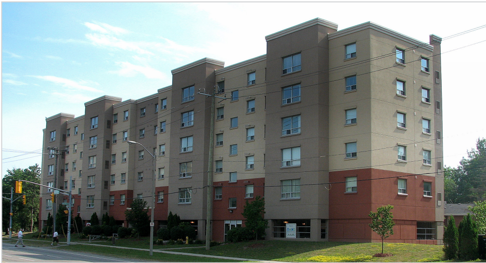
Westcourt Towers - Keats Way, Waterloo, ON
