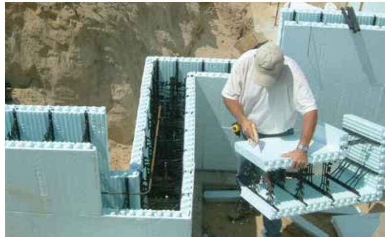
Constructing ICF elements.
