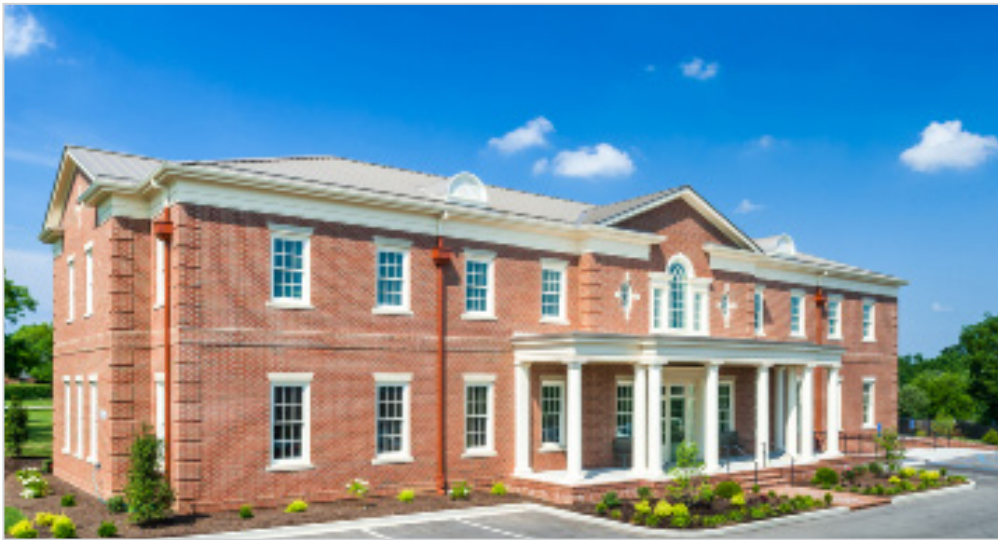
CMTA Office Building - Lexington, Kentucky
